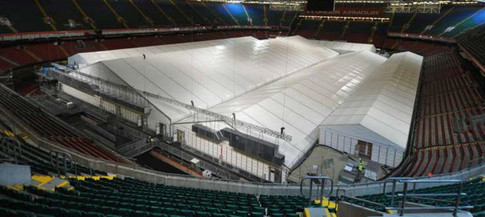
Extensive rigging experience allowed for the hanging of the extremely large steel supply ducting from the stadium's regular roof truss, all to free up valuable floor space, combined with running innovative fabric ducts at 2.5m x 2.5m, neatly threaded through the modular scaffold support grid.
