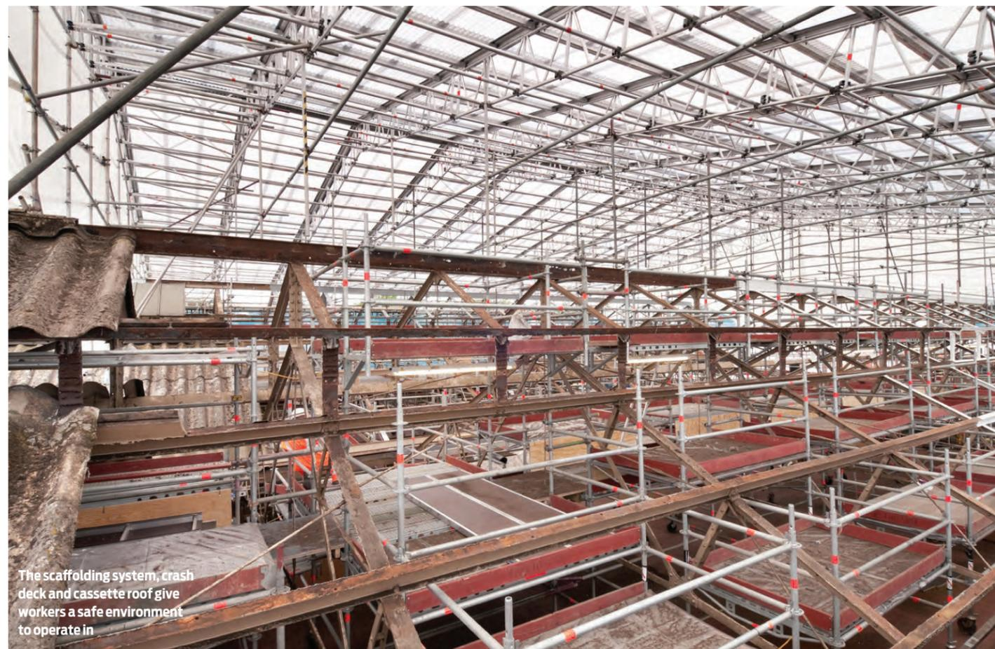
The scaffolding system, crash deck and cassette roof give workers a safe environment to operate in
